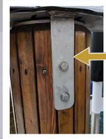
Stainless Steel Piling Double Mount Brackets with Insulator Pad
